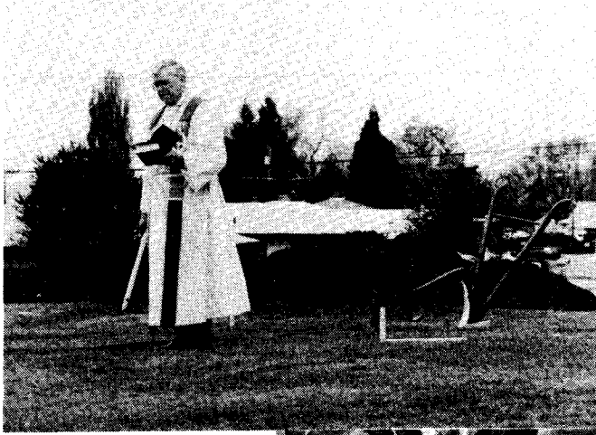
Ground Breaking for New Church at 5520 N.E. Killingsworth Street April 17, 1988
